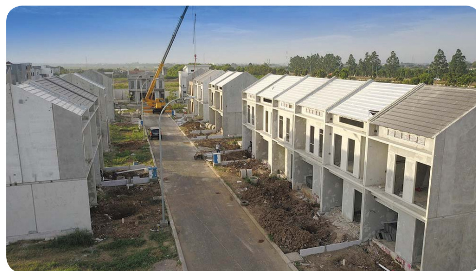
Progress New Shinano Precast.
